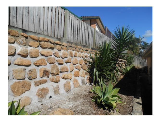
The team at Australian Retaining walls then select the biggest rocks for the base and start building up to 1m in height using the smallest rocks for the caps at the top. As always Australian Retaining walls backfill the wall with 20mm gravel. Outlets are created every metre from 65mm drainage pipe to combat the excessive amounts of rainwater seeping down from the top property. Another satisfied customer for Australian Retaining walls.
