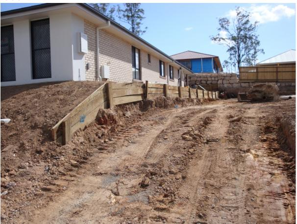
This wall is approximately 27 metres long x 1 metre high. The concrete piers are at 2 metre centres approx 1 metre deep and 450mm wide. The wall is backfilled with 20mm drainage gravel, geotextile fabric and an ag. pipe.
